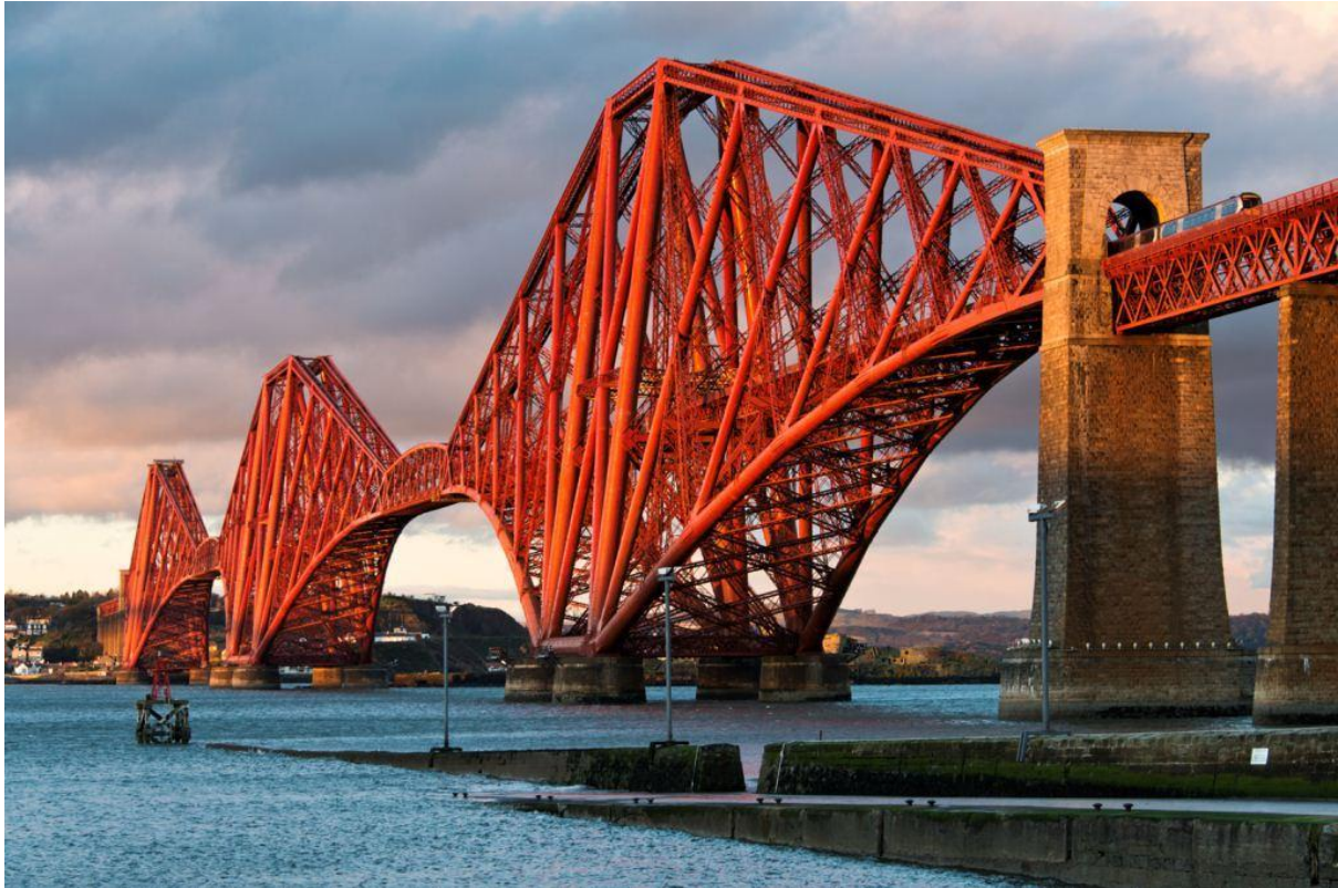
Figure 1: The Forth Bridge after its recent restoration was complete in 2012
