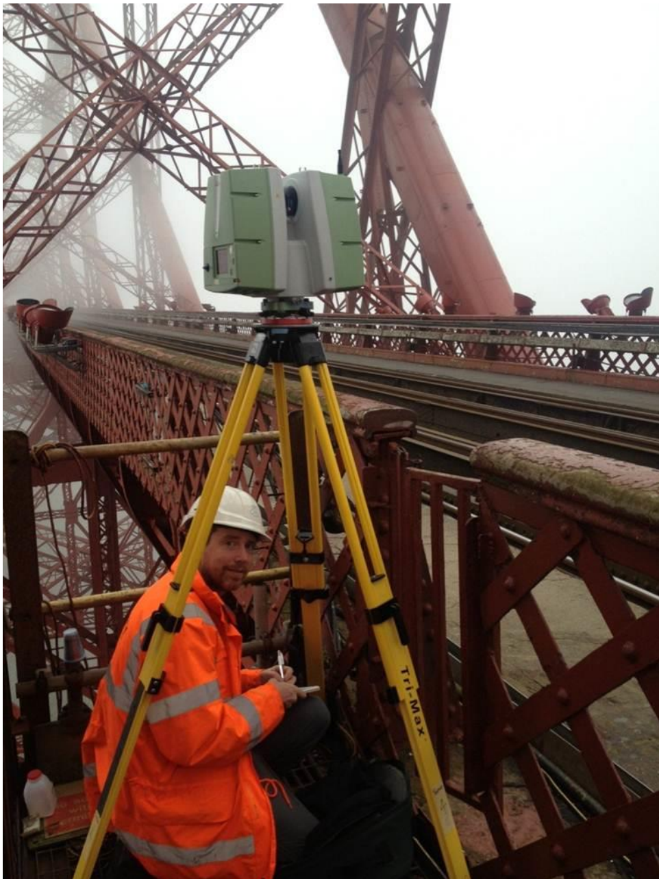
Figure 3: James Hepher of Historic Scotland with a Leica laser scanner. He was one of a team working on a pilot 3D survey of the Forth Bridge in August 2013.
